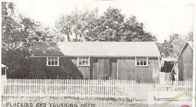
PLUCKING AND TRUSSING SHED
